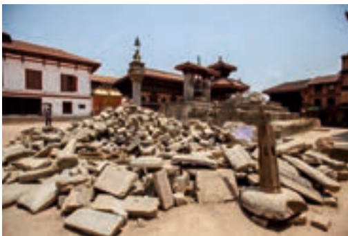
Photo 2: Earthquake damaged Batshala Temple at Durbar Square, Bhaktapur Heritage Site, Nepal (Photo credit: Jitendra Bajracharya)
