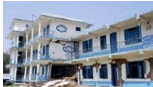
The ruins of a 4 storey tall school in Sangachowk, Sindhupalchowk. The ground floor has collapsed completely! The headmaster told us that, had it been a school day, they could have lost upto 400 children
