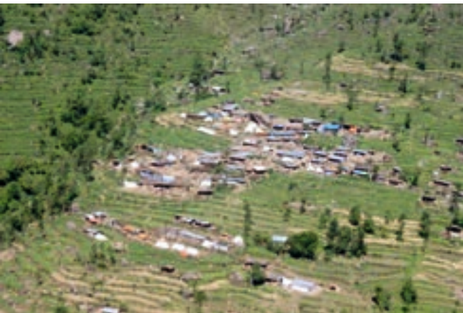
Figure 17. Highly damaged village on old landslide mass in Sindhupalchowk district
