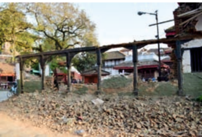
Figure 3b. A Damaged Heritage Site
