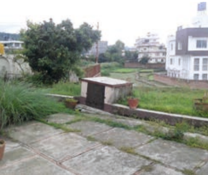
Figure 14. Land subsidence problem in cut -and- fill area of a private house compound in Budhanilkantha, north Kathmandu.
