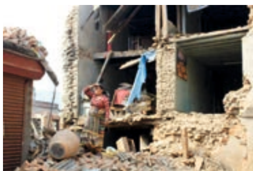
Figure 5. A woman stands in front of partially damaged houses
