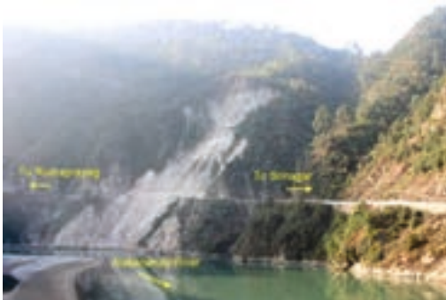
Figure 18. Shallow landslide on old landslide mass observed in Indian Himalaya, a typical example of road side landslide problem in the Indian Himalaya
