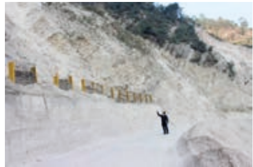
Figure 19. Improper mitigation measure on shallow landslide occurred on old landslide mass in the Indian Himalaya
