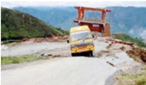
HRDC relief bus navigating a 'caved in' road in the backdrop of an earthquake destroyed resort: Bhotechowr, Sindhupalchowk
