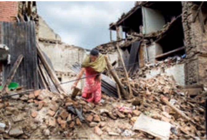
Photo 1: Damaged house near Main Gate at the Bhaktapur Heritage site, Nepal (Photo credit: Jitendra Bajracharya)
