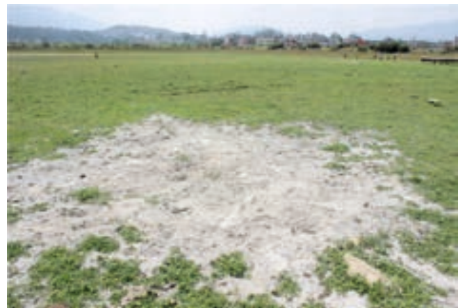
Figure 14. Land subsidence problem in cut -and- fill area of a private house compound in Budhanilkantha, north Kathmandu.
