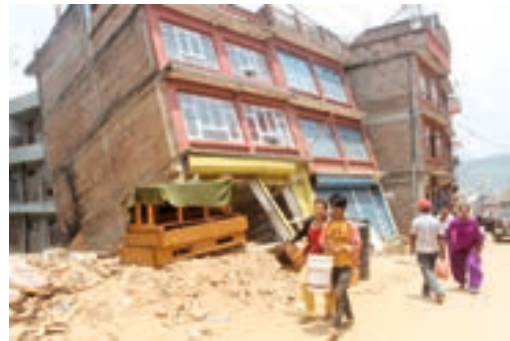
Figure 10. Earthquake damaged houses in Chautara town
